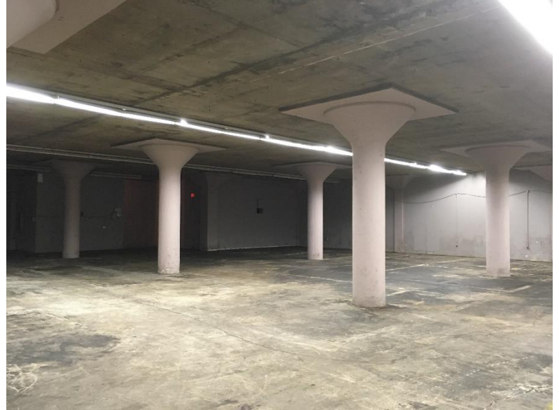
1901 Fairview- Lower Level
